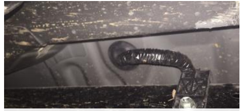
10. locate this grommet below the N/S front door.
