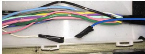
25. Insulate both sections of wire and secure before closing the box.
