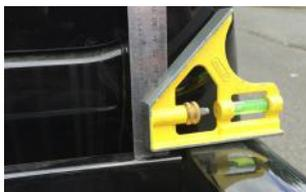
7. Check the level of the bulkhead rail and side rails.
