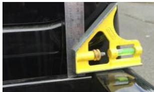
7. Check the level of the bulkhead rail and side rails.
