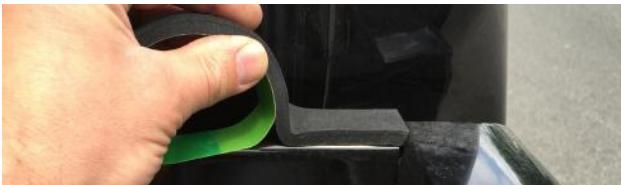
8. If there is a difference apply the self adhesive Neoprene strip (supplied in the fitting kit) to the bulkhead rail. Ensure there are no gaps at the ends.
