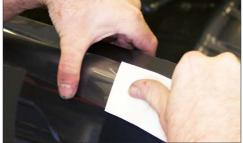
16 Apply it to the tailgate, rubbing outwards to remove any bubbles as you go. 17 Cut the other end square
