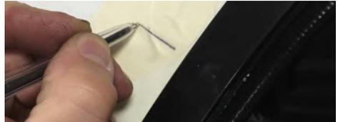
4. Mark the positions of the screws onto the masking tape. This will help locate the positions later.
