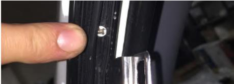
3. Slide open the rear section of the window and locate the fixing screws within the inner channel of the frame.
