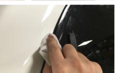
**22.** Use silicone or multi-purpose wipes for the final finish. Check there is a continuous fillet of sealant along the top and sides of the window. If necessary, apply a little more sealant then clean-up using the wipes as before.
