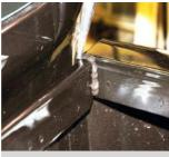
14. Fill the join between the front and side rails with silicone.
