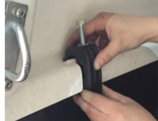
**16.** Tighten the clamps to approx 6Nm.
