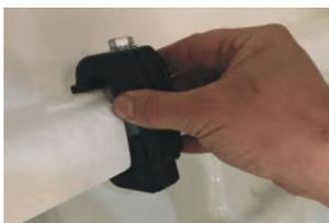
13. Tighten the clamps to 8Nm (start with the front ones. Check them again after 30mis.
