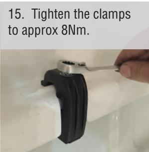
15. Tighten the clamps to approx 8Nm.
