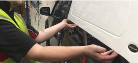
12. Carefully adjust the position of the canopy so that it lies centrally on the vehicle.
