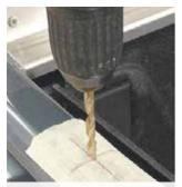
**10.** Drill a 3mm pilot hole 15mm from the inside edge at each mark. Drill again with an 9mm bit.
