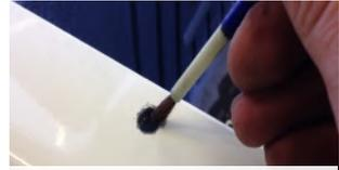
**7.** Remove all swarf and paint hole edges with zinc rich primer to prevent corrosion.
