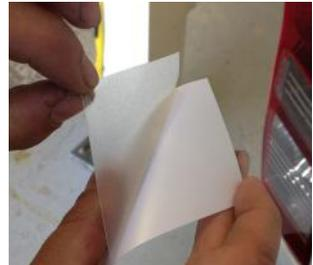
**20.** Partly remove the backing from the tape.
